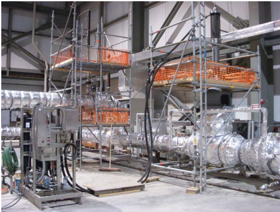
HPA-3000.HV Blow Down Service System for pre- commissioning cleaning of Heavy Duty Steam Turbines (2-3 second operation)
